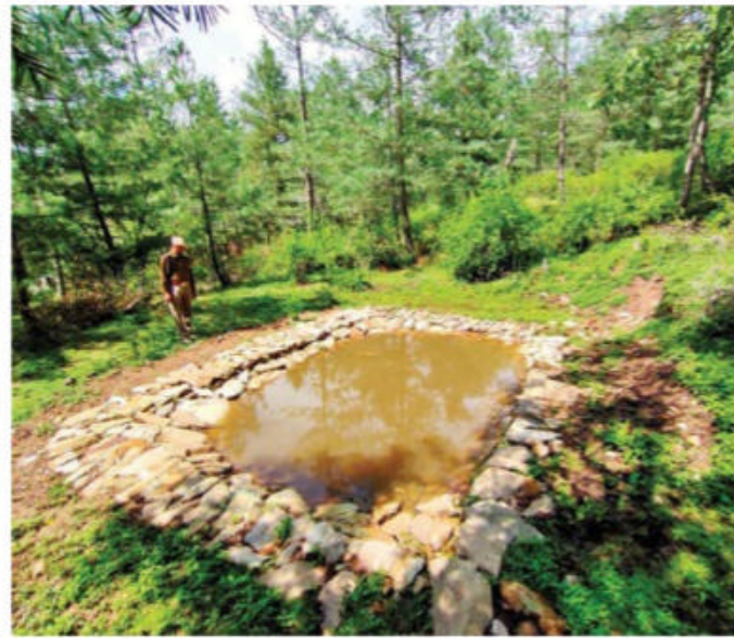
(Left) IFS Officer Vaibhav Singh; (Right) One of the hundreds of chal kahls constructed to harvest rainwater that helps restore the fragile terrain of the Rudraprayag hills.
